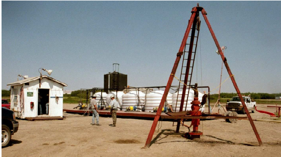
Production and grouting with gypsum-forming solutions at Mosaic Potash Esterhazy Ltd. (Canada)
