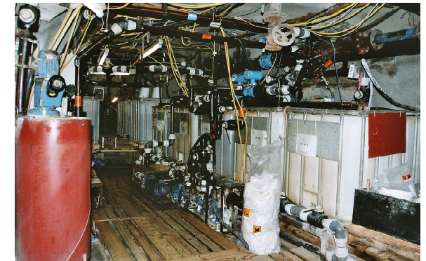
Plant for preparation of \text{BaSO}_4 -forming solution in the former uranium mine Koenigstein (Wismut GmbH)
